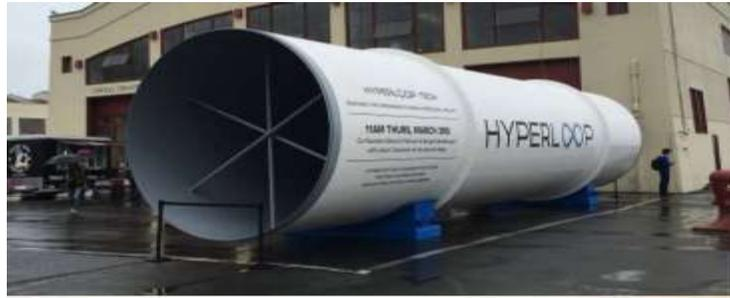
The tube is made of steel. Two tubes will be welded together in a side by side configuration to allow the capsules to travel both directions. □ Pylons are placed every 100 ft (30 m) to support the tube. □ Solar arrays will cover the top of the tubes in order to provide power to the system. □ Tubes are made by the new material ‘VIBRANIUM’.
