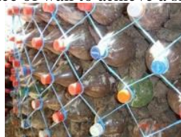
Figure 16: Plastic bottle necks tied together to keep bottles in place Figure 17: Wall being plastered
