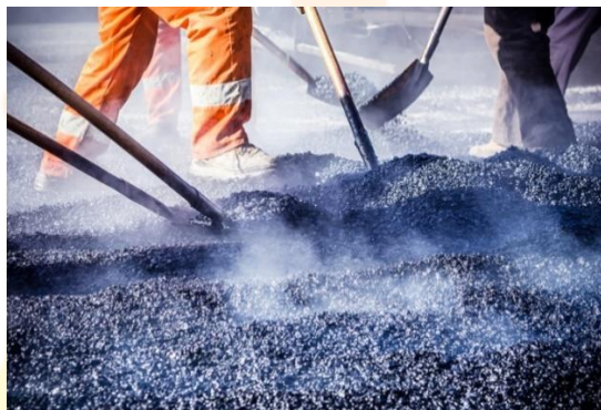
Fig. 3: Hot-Mix Asphalt Patching
