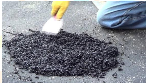
Fig. 2: Cold-Mix Asphalt Patching
