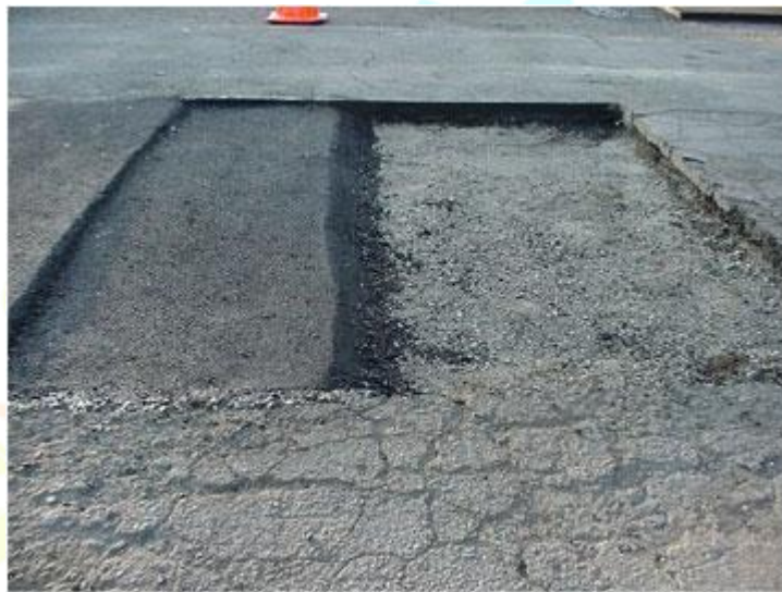
Fig. 5: Full-Depth Patching
