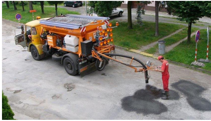
Fig. 4: Spray Injection Patching
