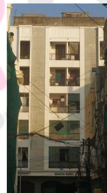
Fig.4 West Façade of the building as viewed from the street.
