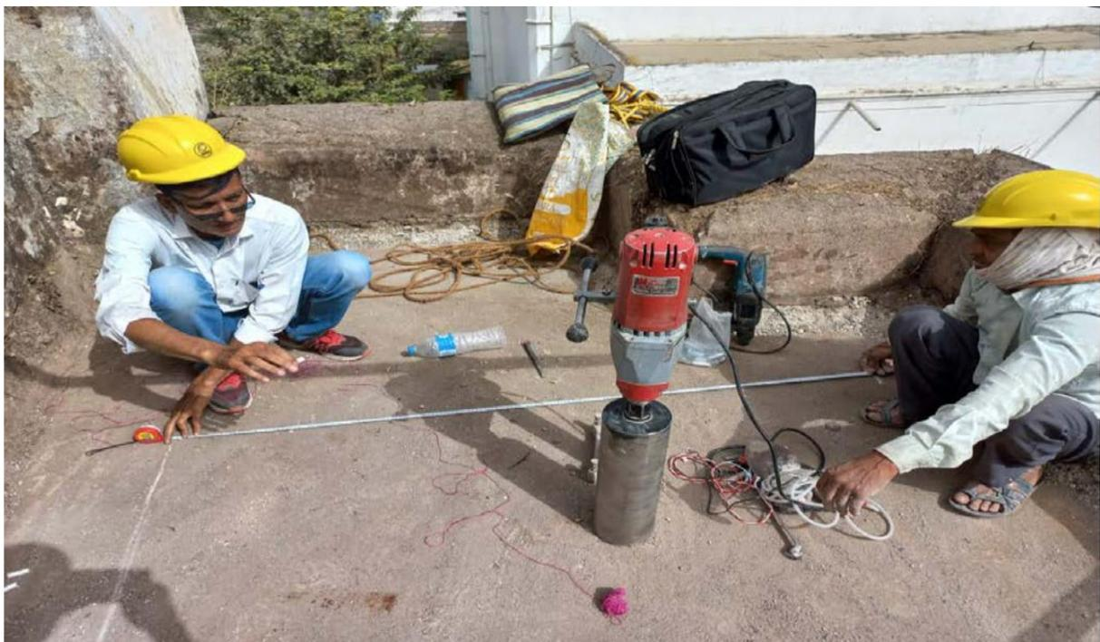
**Fig No:-3.4 inserting grouting sully**
