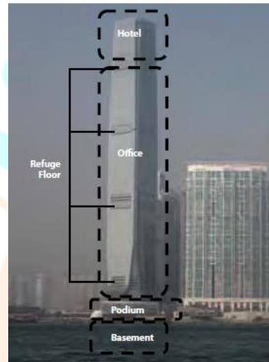
FIGURE 13. Different zoning orders of the fire detection system in super tall buildings B. [11]
