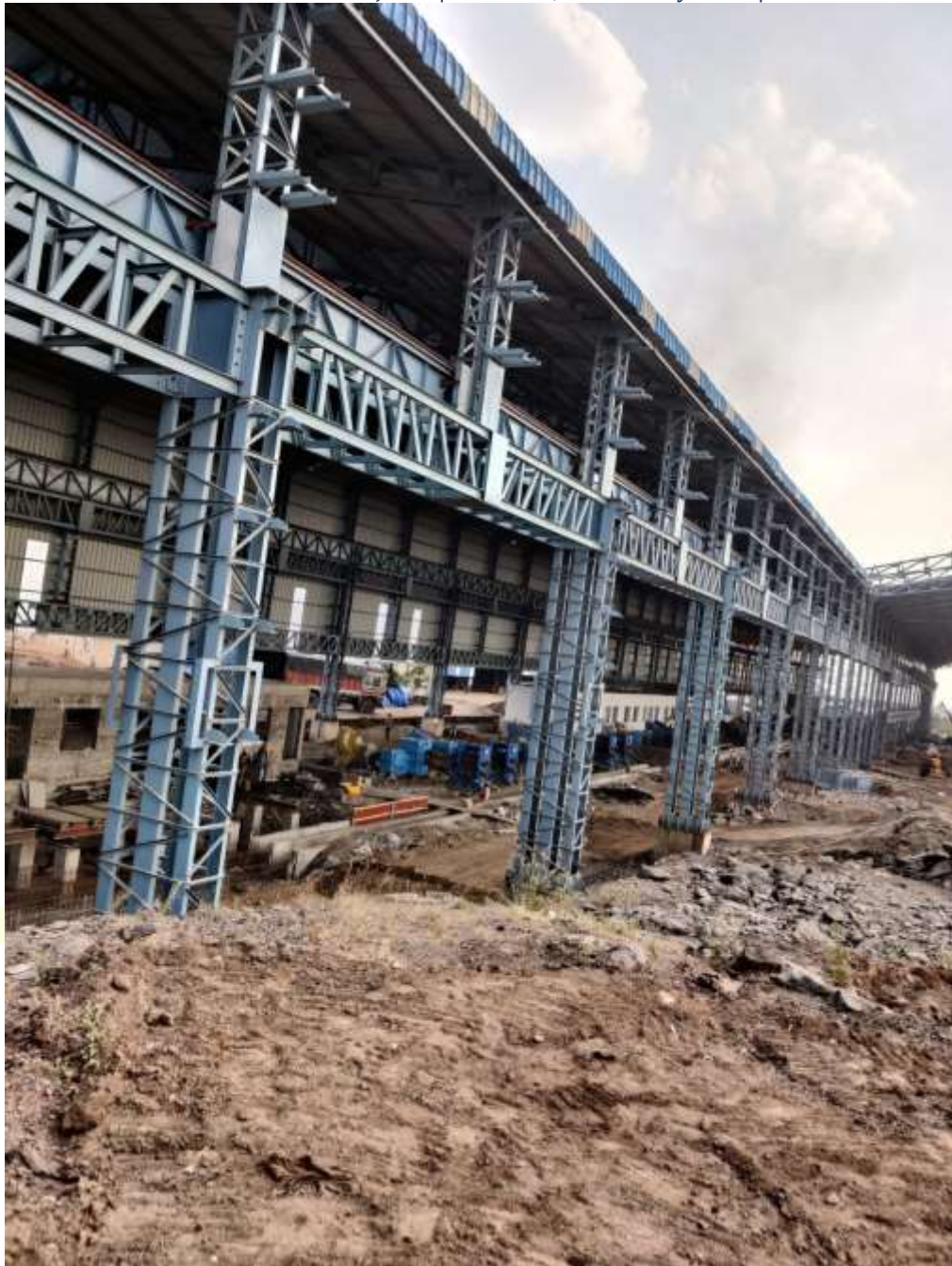
Figure 1.5: Structural Fabrication of beam column framing of one of the industrial Condition around plinth level
