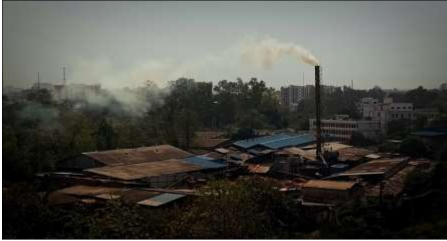
Fig.1: Air Pollution from stack
