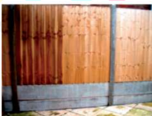
Figure 4.21 Protection of Fence Base with Impermeable material.
