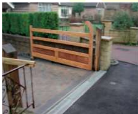
Figure 4.20 Property Boundary Wall and Lower Sealed Gate
