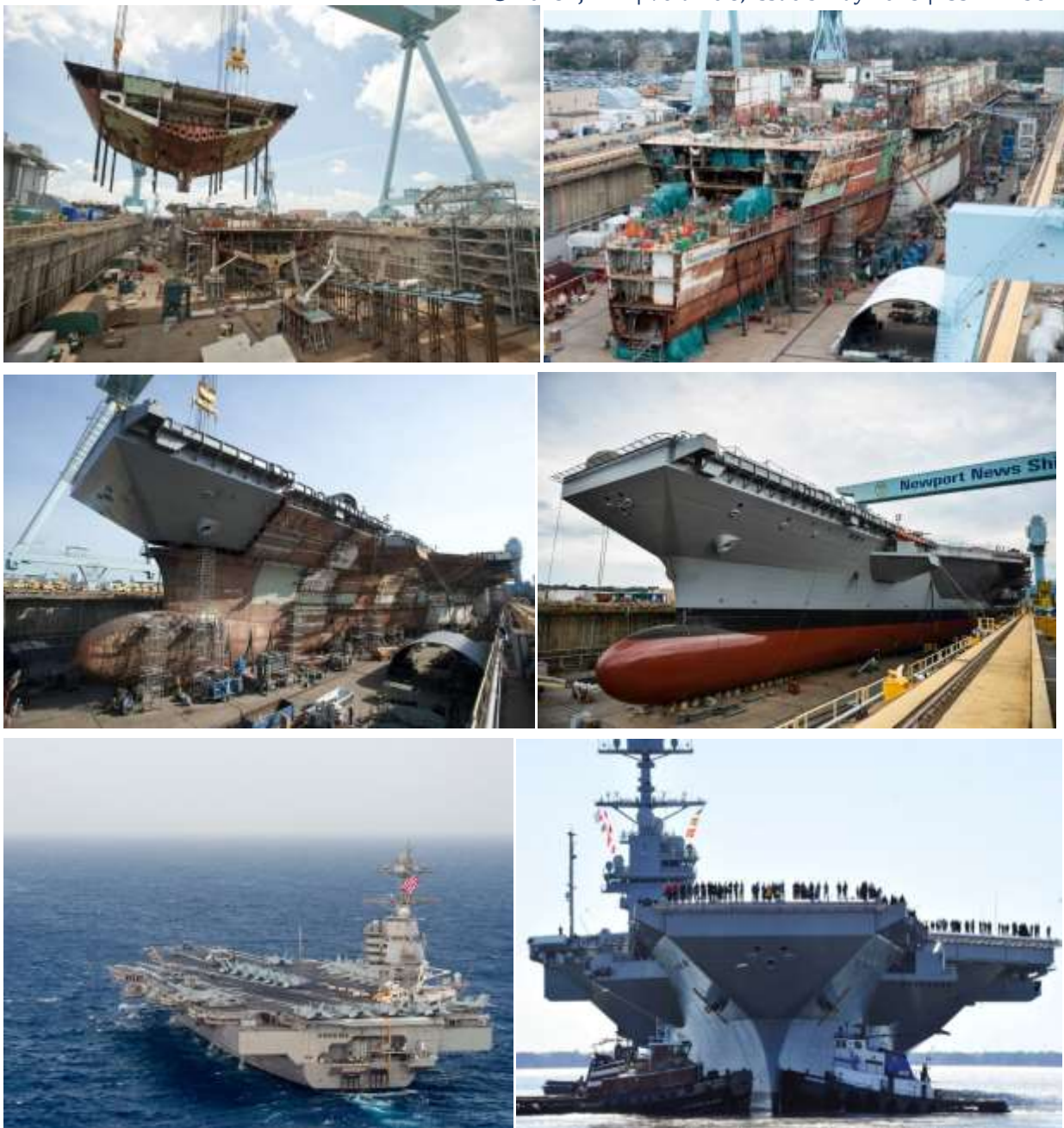
Figure 6: Construction stages and images of the latest nuclear powered aircraft carrier Gerald R. Ford(CVN 78) for US Navy 60
