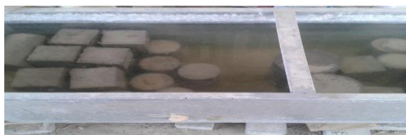
Figure-02 Curing of concrete Moulds
