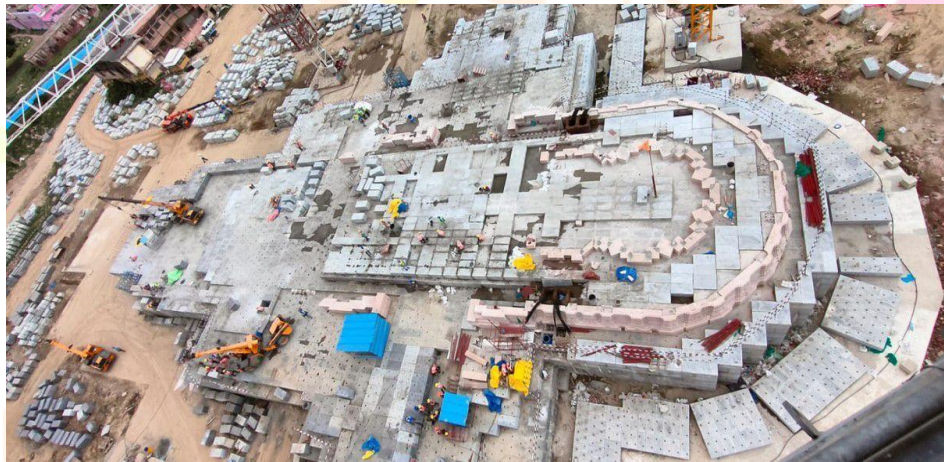
Main construction site Ram Mandir Parisar
