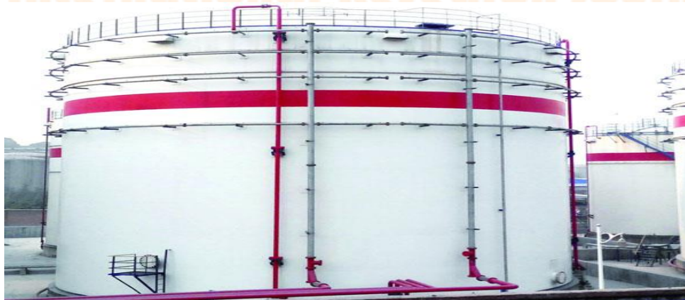
Fig.1 Water storage tank
