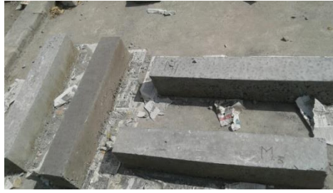
Figure: 3.14 Casting of Beam
