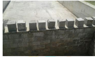
Figure: 3.12 Casting of Cubes
