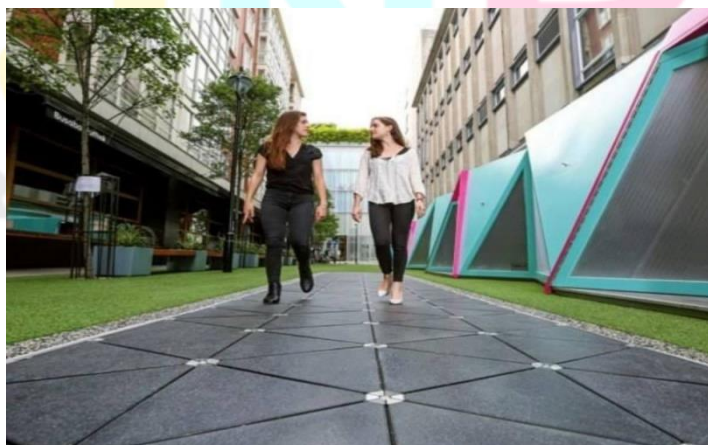
fig.3.4. Kinetic paving in the street
