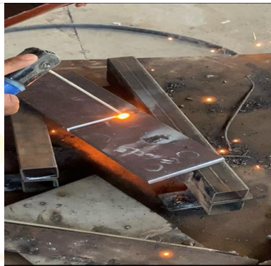
Fig 2.4 Arc Welding MS Plate
