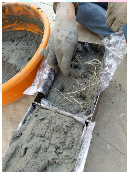
Fig 3.1 C-2 Placing of sisal fiber in zig zag manner
