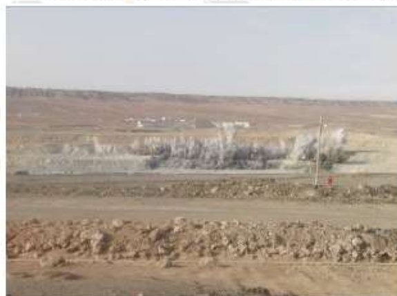
(c) Blasting site 1
