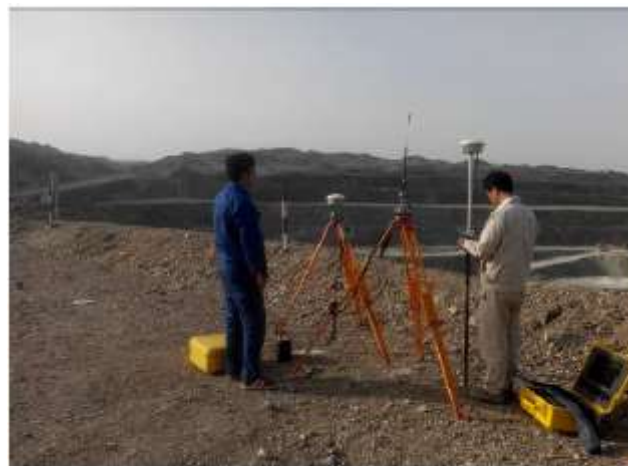
(a) Survey point setting out
