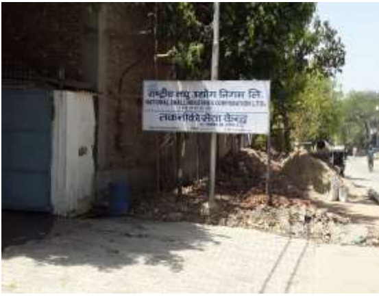
Figure 8: Front view of NSIC
