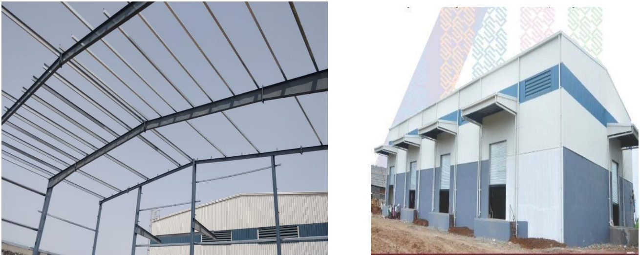
Fig1.Structural frame and warehouse
