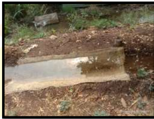
Fig. 7) Canal Lining By innovative method
