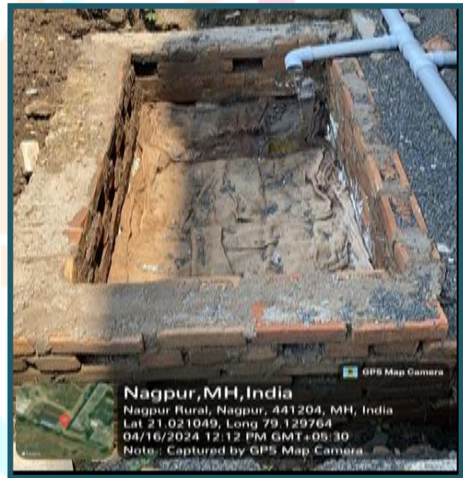
Figure 03: Constructed Magic soak Pit
