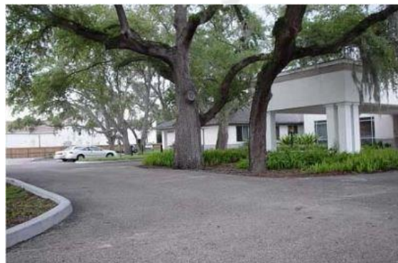
Figure .1 Porous Concrete Road
