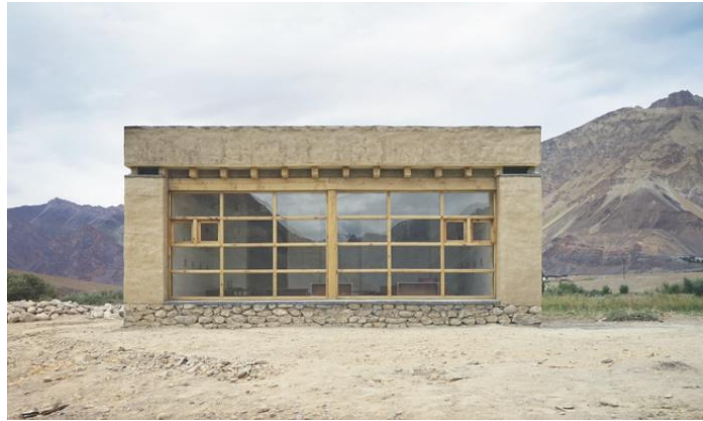
Figure 4: The Upper Wall Structure Is Built Of Two Layers Of 30cm Sun-Dried Mud Bricks, With Locally Sourced Straw Insulation Between.
