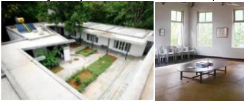
Figure 9 : Windows provide for cross ventilation at Rishi Valley school
