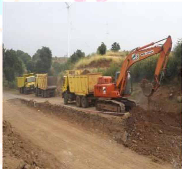
Image:- Site Excavation
