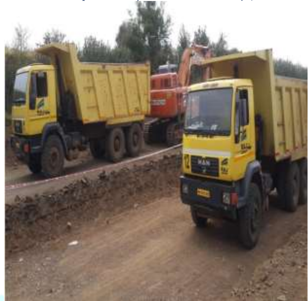
Image: - Site Excavation
