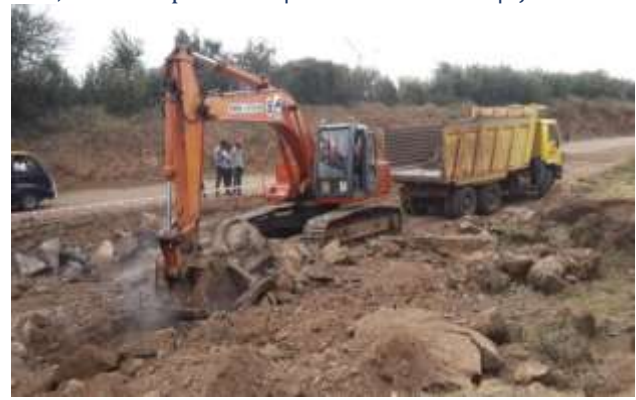
Image: - Site Excavation
