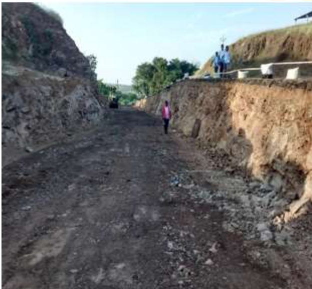
Image: - Site Excavation
