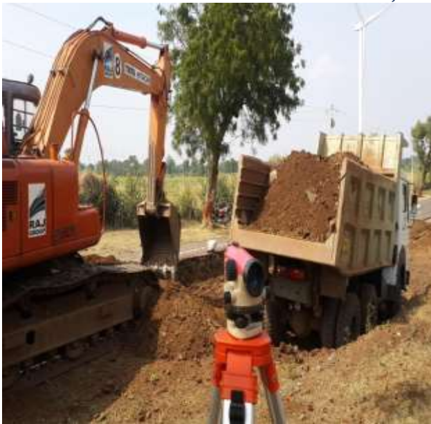
Image: - Site Excavation
