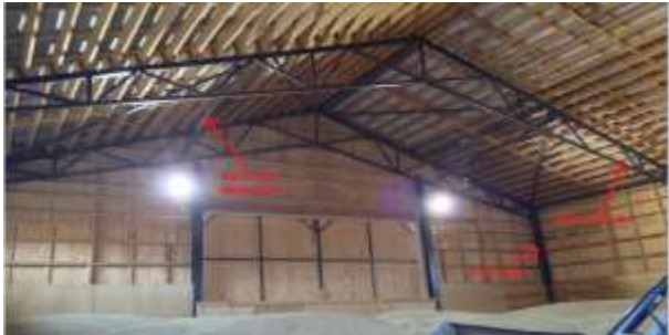
Fig 2: the interior of a warehouse building
