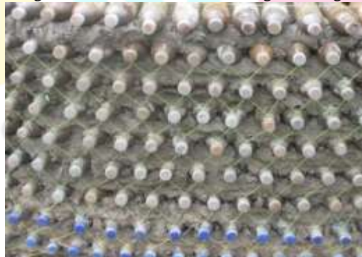
Fig 2 Plastic Bottle As brick
