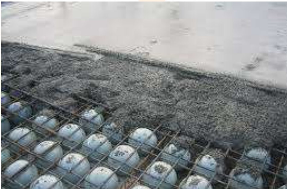
Fig. 1 Bubble deck slab
