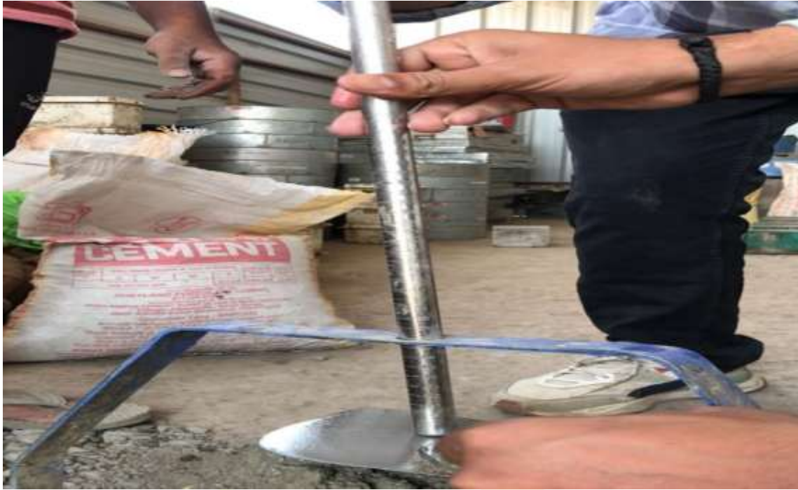
Fig.9 Taking slump test measurement
