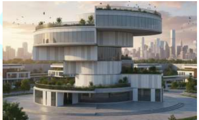
Figure 5. View of the Structure
