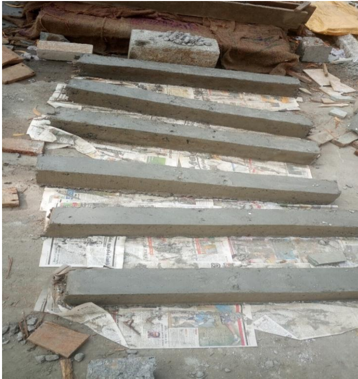
Figure 5.5 Casting of Beams
