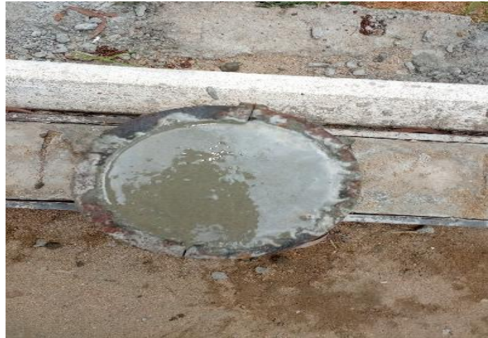
Figure 5.4 Casting of Cylinder
