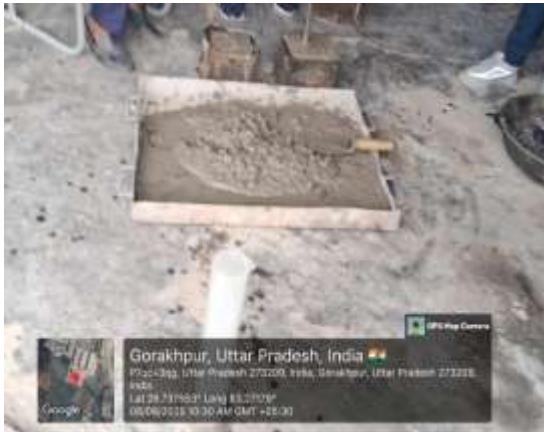
Fig.4. Preparation of bacterial concrete.
