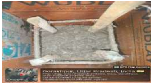
Fig: Casting of BRC
