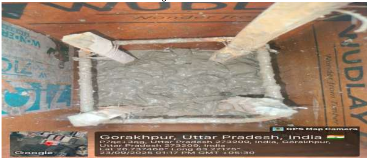
Fig: Casting of BRC
