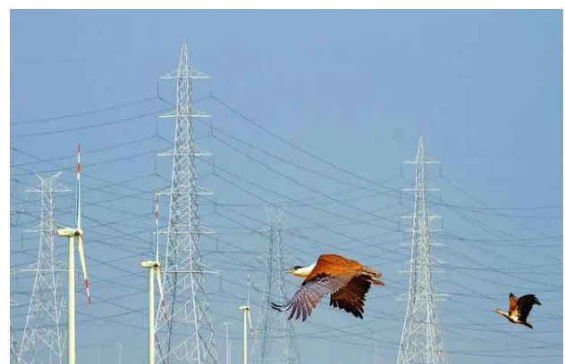
Fig-3: Grid lines hazard for birds
