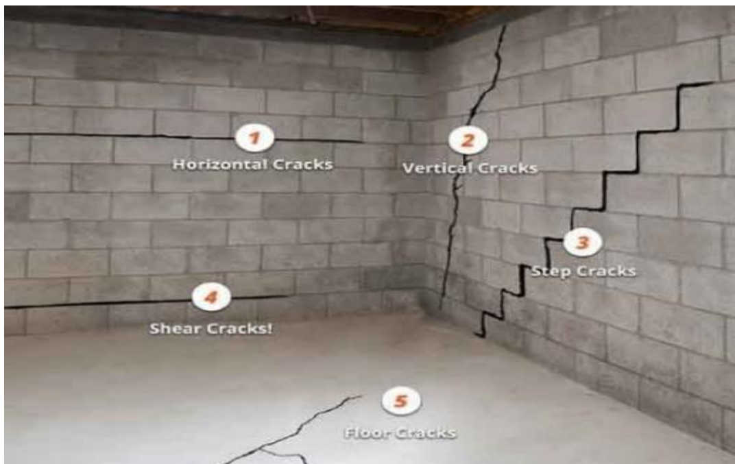
Figure 1.1 Types of Cracks
